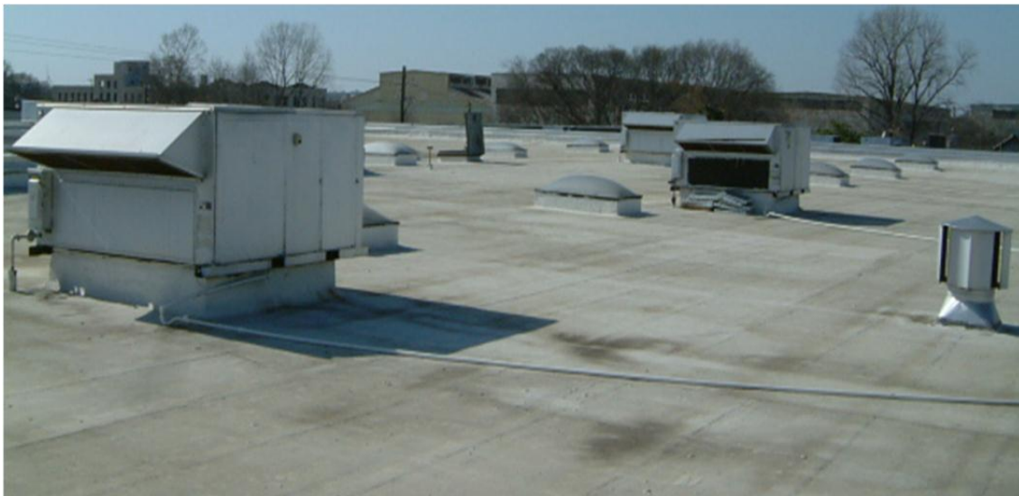
Figure 1) – Typical low-sloped insulated roof
