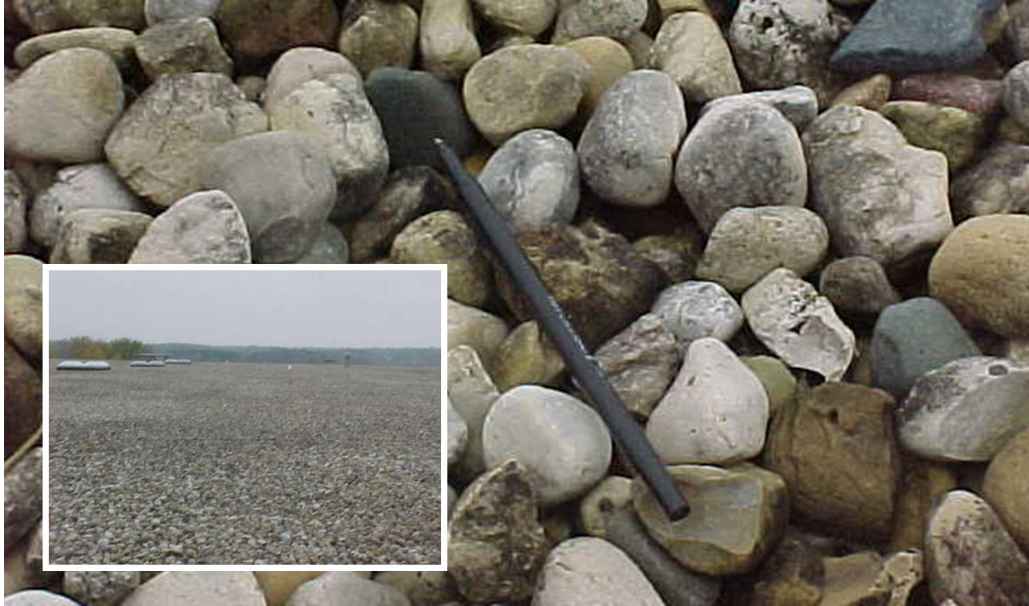
Figure 10) – Visual images of a heavily ballasted EPDM roof
