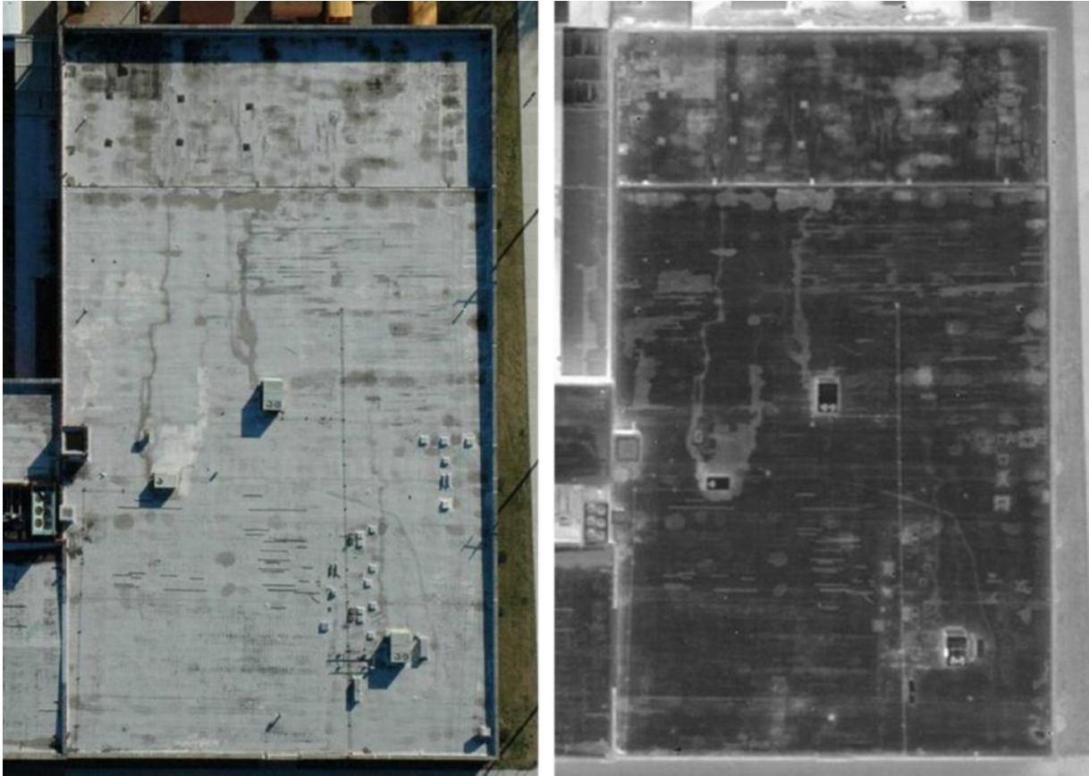
Figure 11) – Visual and thermal aerial images of a stained, worn roof with a highly reflective coating (false apparent wet areas are less reflective)
